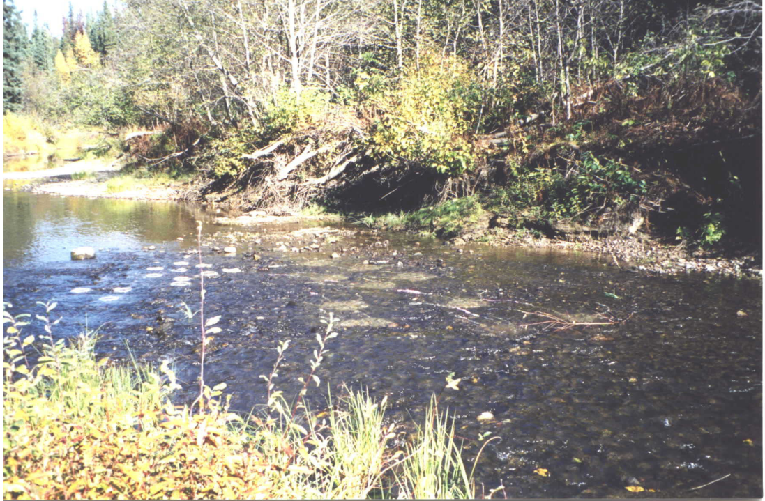
Figure 16 - Infiltration bags should be installed upstream of gravel buckets.
