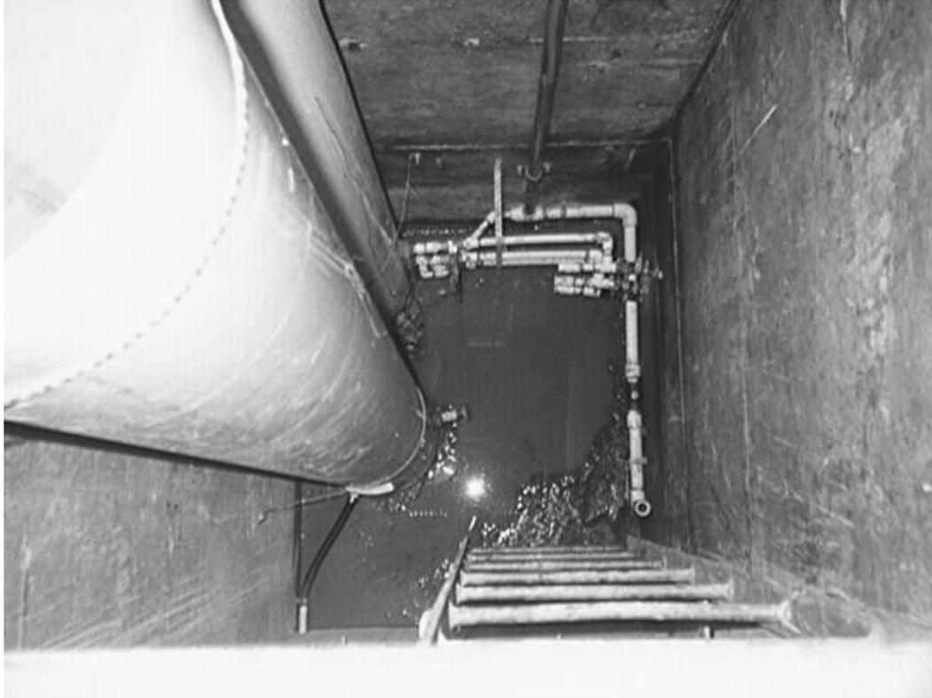
Note: the shelter for this type of installation requires a minimum floor area of 7.5 m<sup>2</sup> (dry well floor area, assuming a 0.31 m diameter wet well, must be at least 1.5 x 2.0 m). The dry well must be fitted with a ladder bolted to the wall, a 37.5 mm floor drain and covered with a trap door or removable floor plates.
