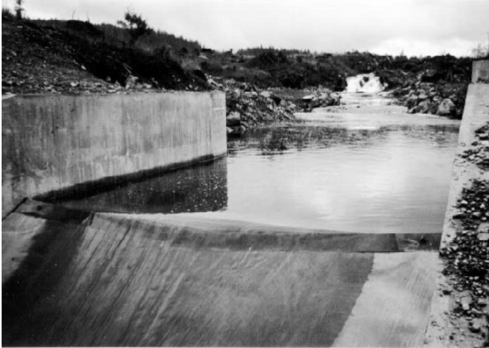
**Figure B-2. Pool formed by a modified Crump Weir, where both a digital and an analogue recorder are installed. Judge Creek, Victoria Water Board. The crest has been formed with a shallow vee to increase low flow sensitivity.**
