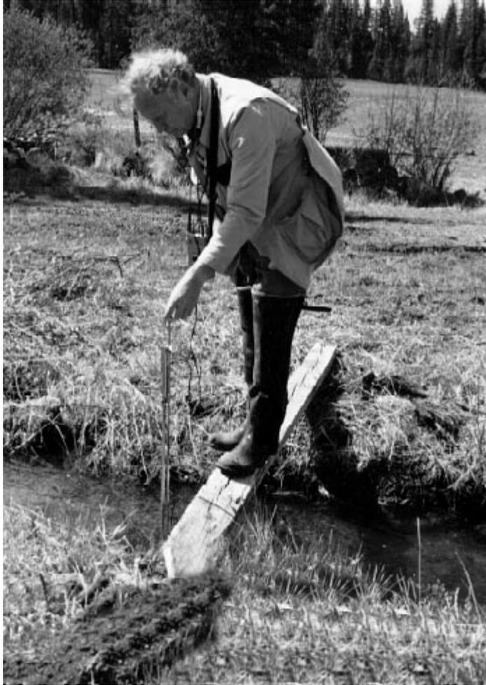
**Figure D-2. Ditch flow measurement using planks.**
